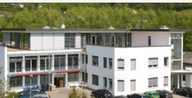
Factory (1.100 m 2 ) in Mittenaar-Bicken (SMD assembling and Production)
