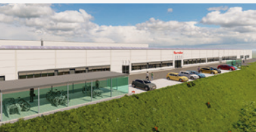
Production and Warehouse (11.000 m 2 ) in Bischoffen
